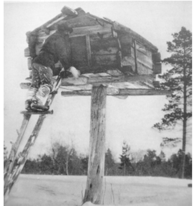
Old storehouse "nili" on the top of a pillar as visual references for design. Photo. Itkonen 1929
