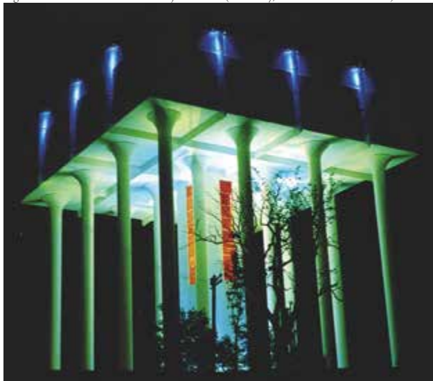
Figure 2: Cranhill Water-tower Project – after (Courtesy, Collective Architecture)
