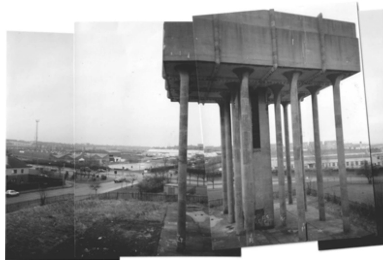
Figure 1: Cranhill Water-tower Project – before (Courtesy, Collective Architecture)
