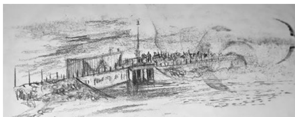
Figure 3. The dam at Porttipahta Reservoir. Brown 2024
