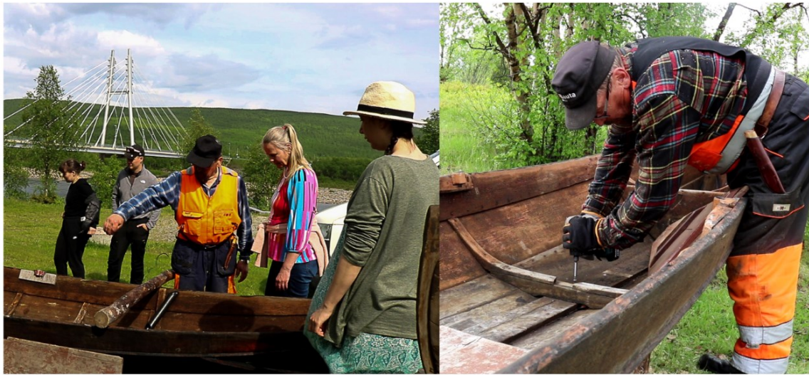
Figure 9. Constructing “Have a Seat”. Photos by Falguni Mazumder, 2024.
