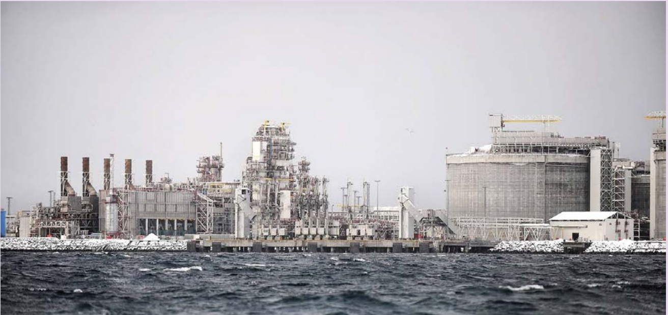
Picture 6.2: State-of-Art Technology in Arctic Conditions: Melkøya LNG Production.
